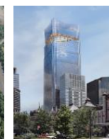
Torch Tower (Building B)
