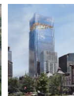
Torch Tower (Building B)
