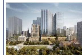
South Tower in South block
