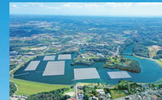
Yamakura Floating Mega Solar Power Plant in Chiba Prefecture
