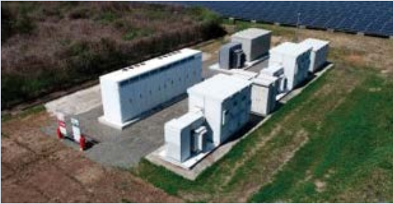
Storage batteries installed at the Kumamoto Arao Megasolar Power Plant
